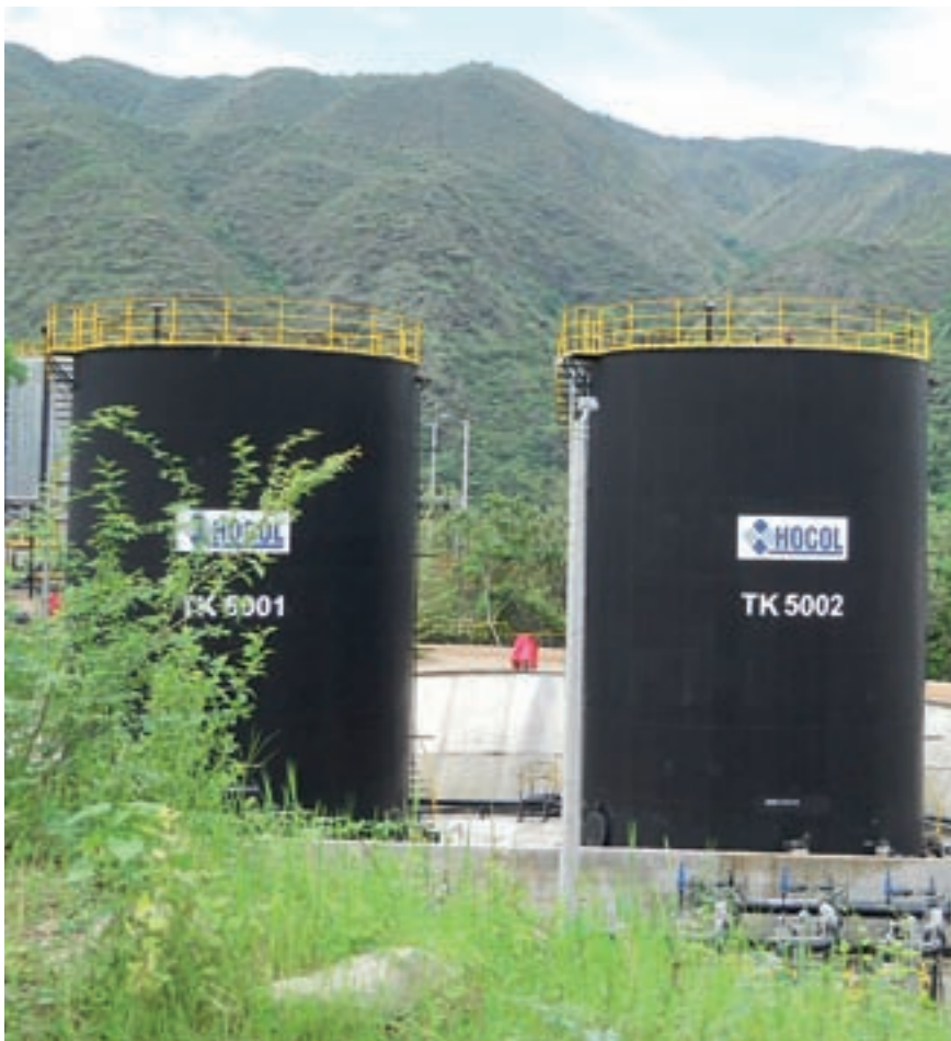
Hocol oil tanks
