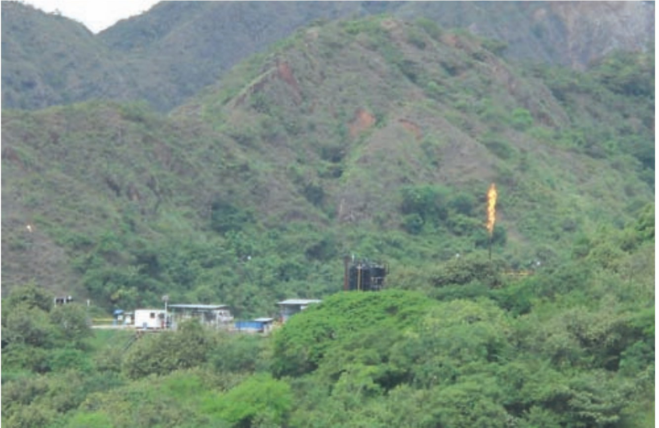
Hocol plant in la Hocha, Colombia
